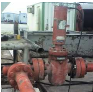
شکل 7: Automatic Choke
